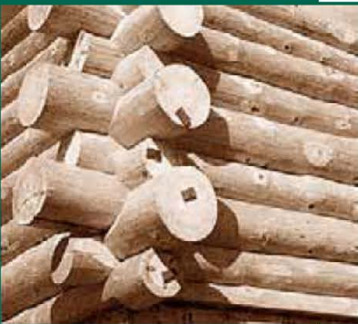
Figure 5-7: Log wall construction
