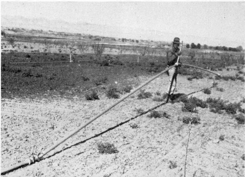
Figure 1.—Moving 2-inch sprinkler line in newly planted peach orchard. The margin between the wet and dry ground is plainly visible.
