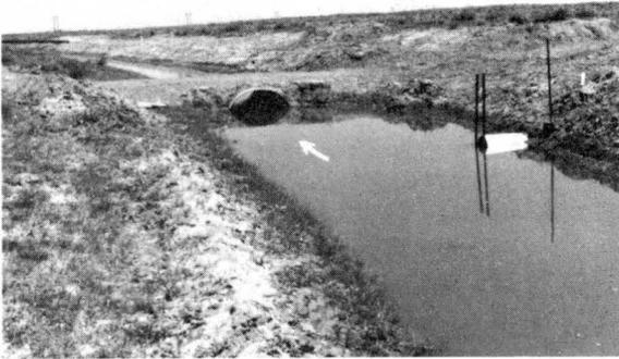
Figure 1. Sand Hill Lateral with Culvert and 12-inch PVC pipe.
