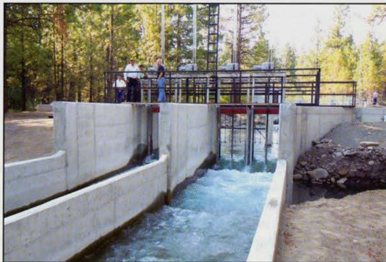
Stakeholders visited a new headgate at the Three Sisters Wychus Creek diversion in Oregon.
