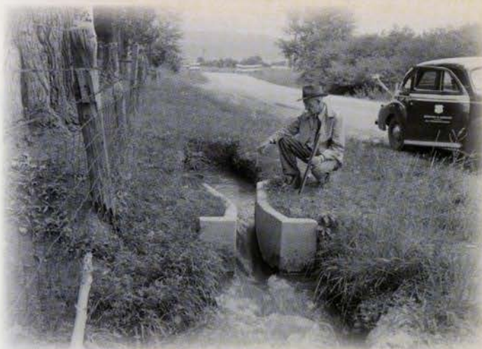
Ralph Parshall poses with a Parshall flume.
