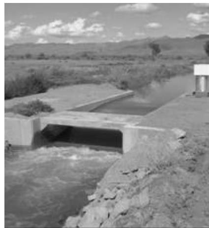
Figure 2. Flow measurement flume at TCID.
