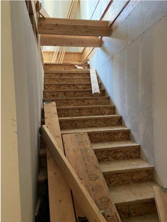
Figure 20 Building 600, onsite wood construction - wood stairs.
