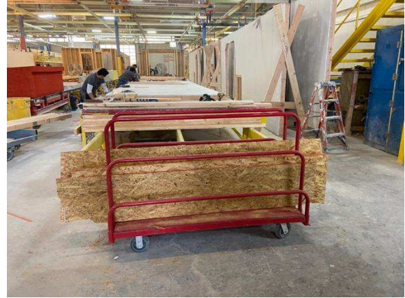
Figure 17 Plywood scraps are collected to be repurposed within the project (March 2023).
