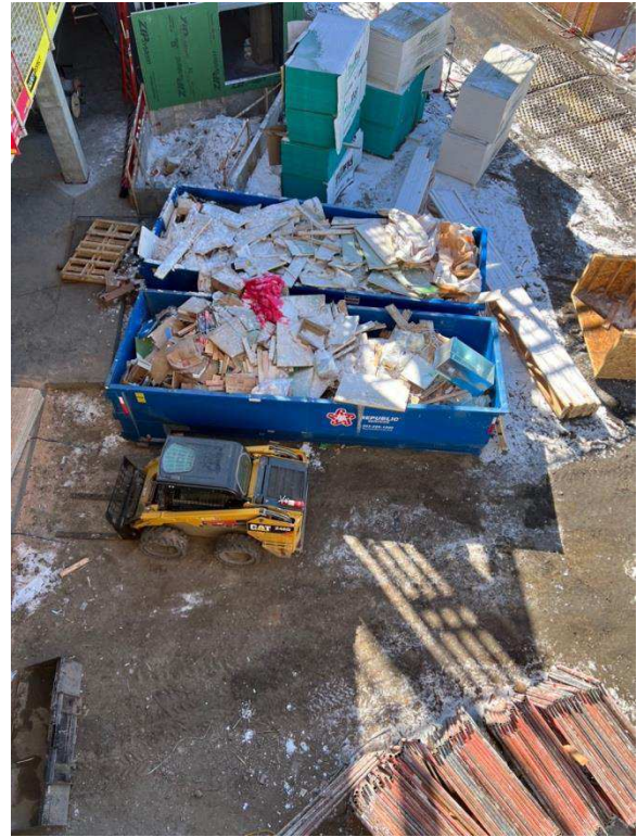
Figure 12 Waste sorting on site-built project (March 2023).
