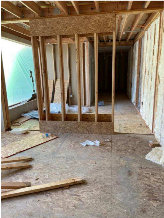
Figure 21 Unquantified wood waste - interior wall required for transport, will be removed.
