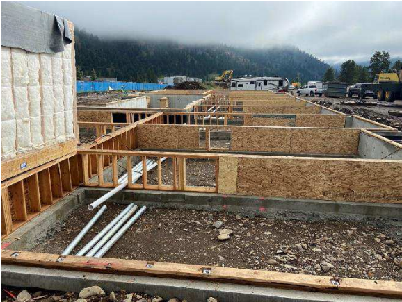
Figure 19 Building 700, unquantified wood framing in basement and crawl space.
