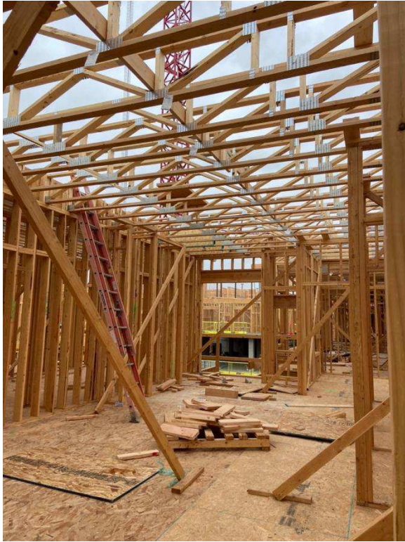
Figure 11 Wood framing waste on site-built project (March 2023).
