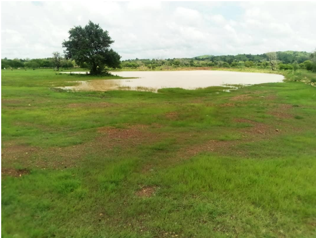
Figure 7. Savannah's dam embankment and water level in mid-August 2022.
