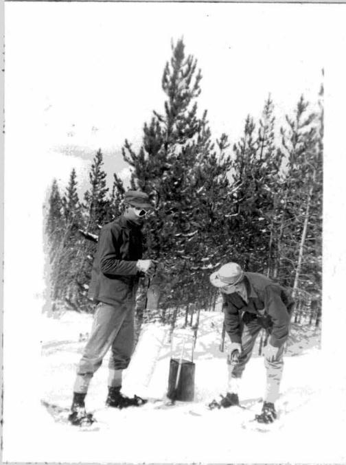
Figure Seven - Weighing a modified Weather Bureau gage to determine the amount of snowfall for the previous week.
