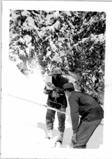
Figure Six - Obtaining the weight of a snow tube and snow core using a Chatillon balance fitted with a cradle.
