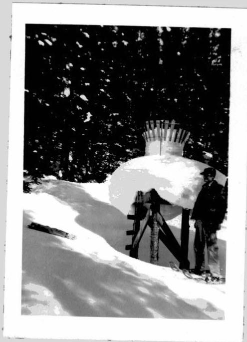
Figure Two - A Sacramento gage fitted with an Alter snow shield. This gage, at 10,000 feet elevation, is a source of data used in forecasting streamflow for the Colorado River.
