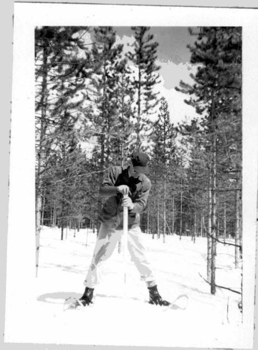
Figure Four - The snow tube is held vertically and is forced into the snow pack smoothly and steadily.
