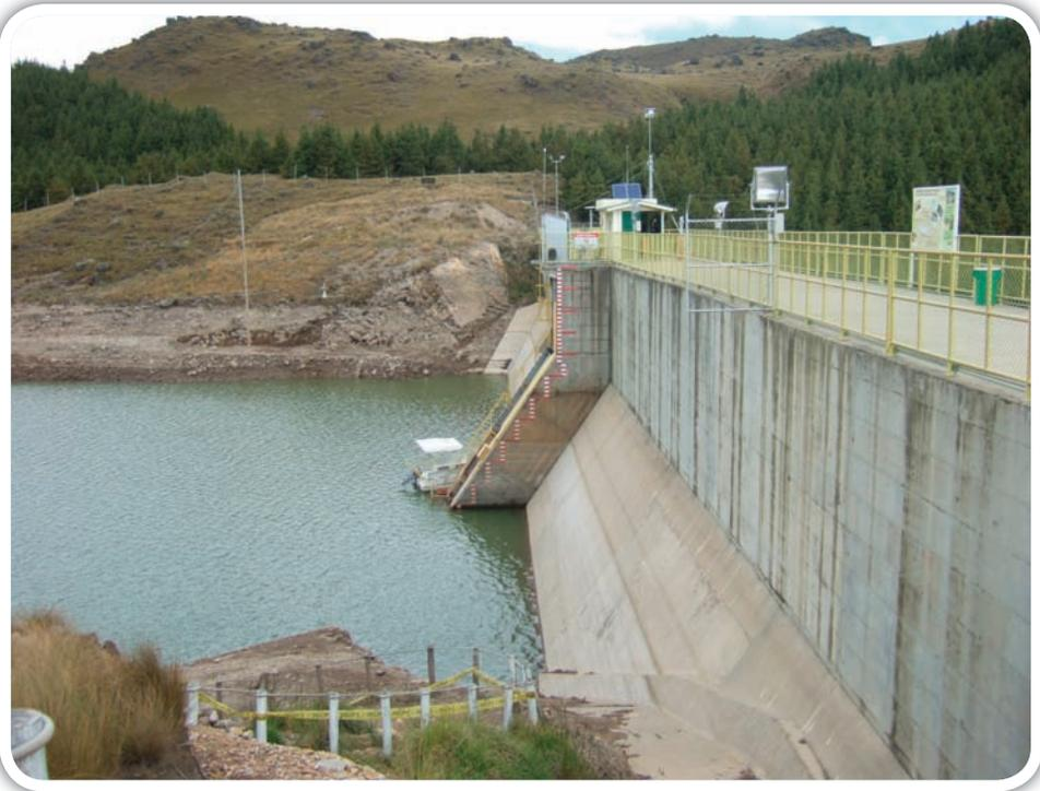
*The Rejo Dam was constructed as part of the effort to control increasing sediment accumulation resulting from mining operations in the Mashcon Basin.*
