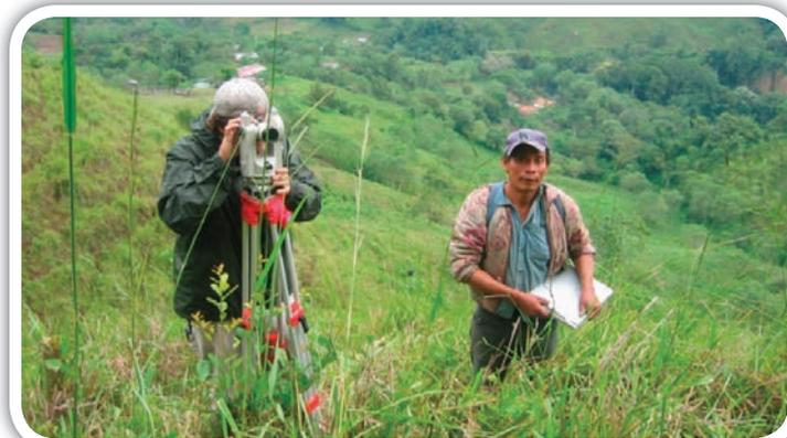
Ben Latham performs a topographic survey in the community of Aldea Nueva, Copán Ruinas, using theodolite equipment for subsequent system design.
