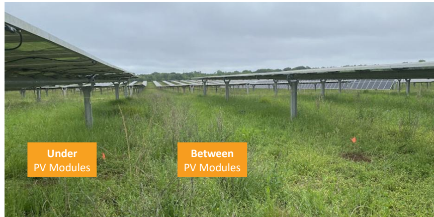
Figure 4. “Zones” relative to PV modules in which vegetation productivity is measured and reported across studies (Table 2). This image illustrates these zones in a single-axis tracking system, however the same concepts are commonly applied in fixed-angle systems as well. Several studies included in Table 2 present array-level biomass data, which in some cases is an average of zones within the array (Andrew et al., 2024; Sturchio et al., 2024) but in other cases, sampling locations relative to the PV modules are not specified (Kampherbeek et al., 2023; Weselek et al., 2021).
