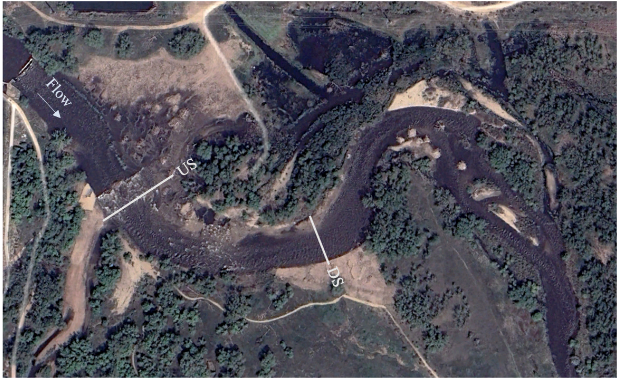
Figure 5. Locations of pebble counts overlain on a 2023 (post-construction) aerial.
