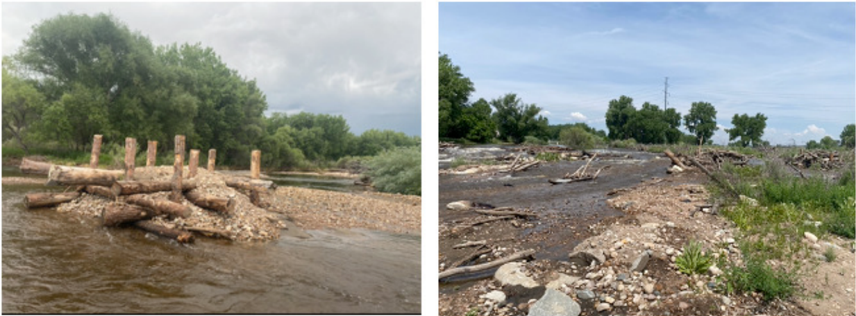
Figure 3. Left: Downstream log structures. Right: Upstream log structures.
