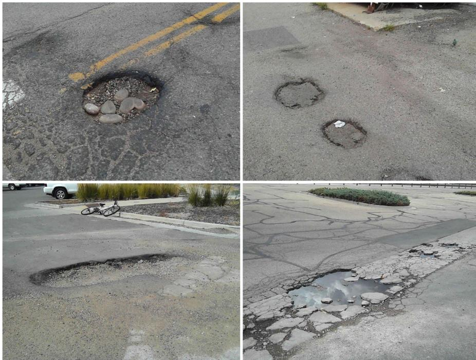
**Figure 1.1:** Samples of potholes.
