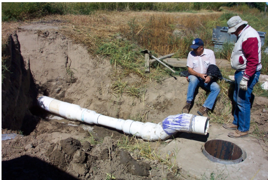
Figure 3. PID Ditch Rider Dennis Waggoner (l) and Ditch Superintendant Dan Korf (r) assisting with the May, 2003 pipe-fitting Venturi demonstration site installation
