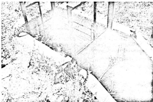
Figure 1.--Field installation of constant-head-orifice farm turnout. The orifice gate is in the center of the photograph and the turnout gate at the upper left. Flow is from right to left.
