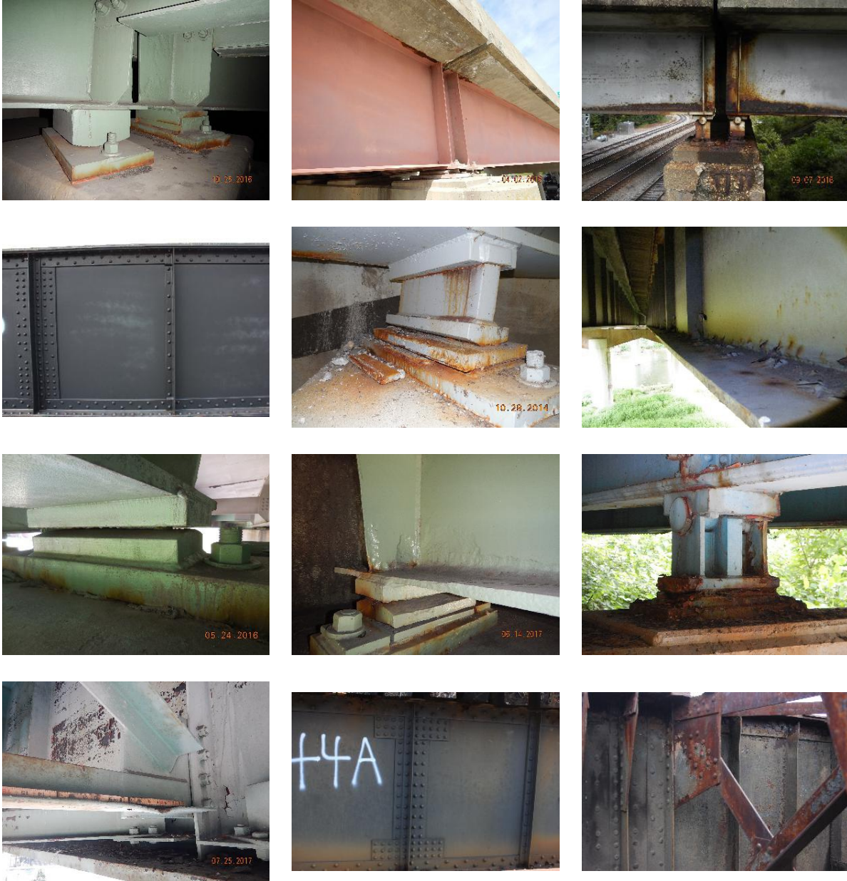
Figure 3.52: Sample full-sized images for the identification of steel bridge connections [1]
