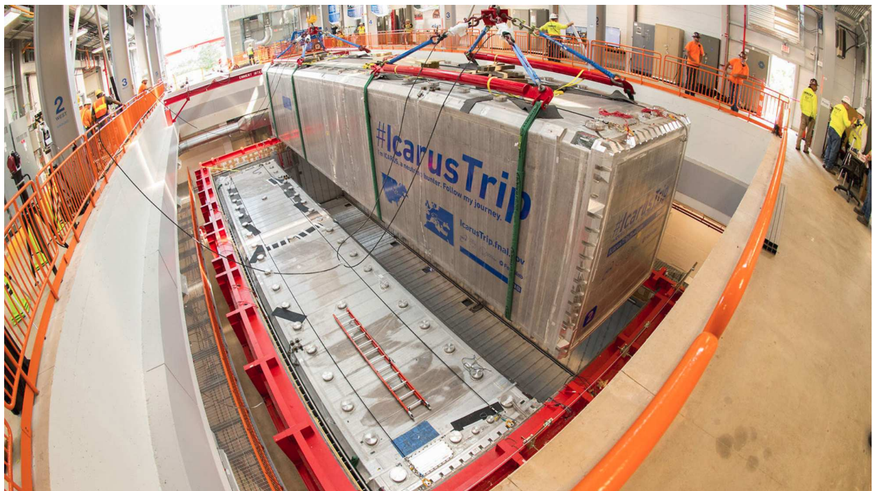
Figure 2.3: A ICARUS T-300 module being lowered into the warm vessel in the Short Baseline Far Detector building at Fermilab. Photo from Fermilab Creative Services.
