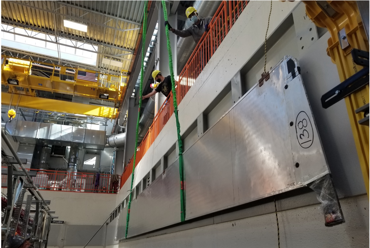
Figure 4.10: A MINOS module being lowered by technicians for the East-North Side CRT wall.
