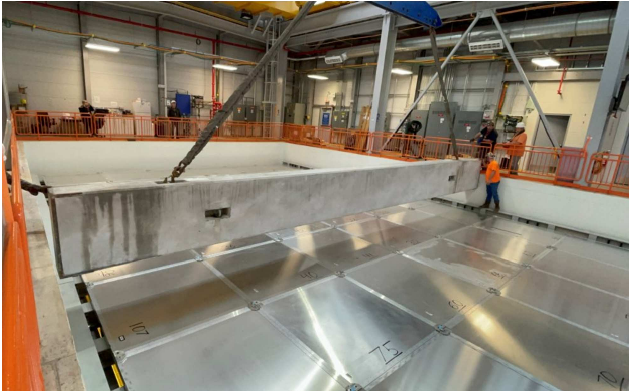
Figure 2.7: First block of first layer of concrete overburden being installed above the ICARUS Top CRT.
