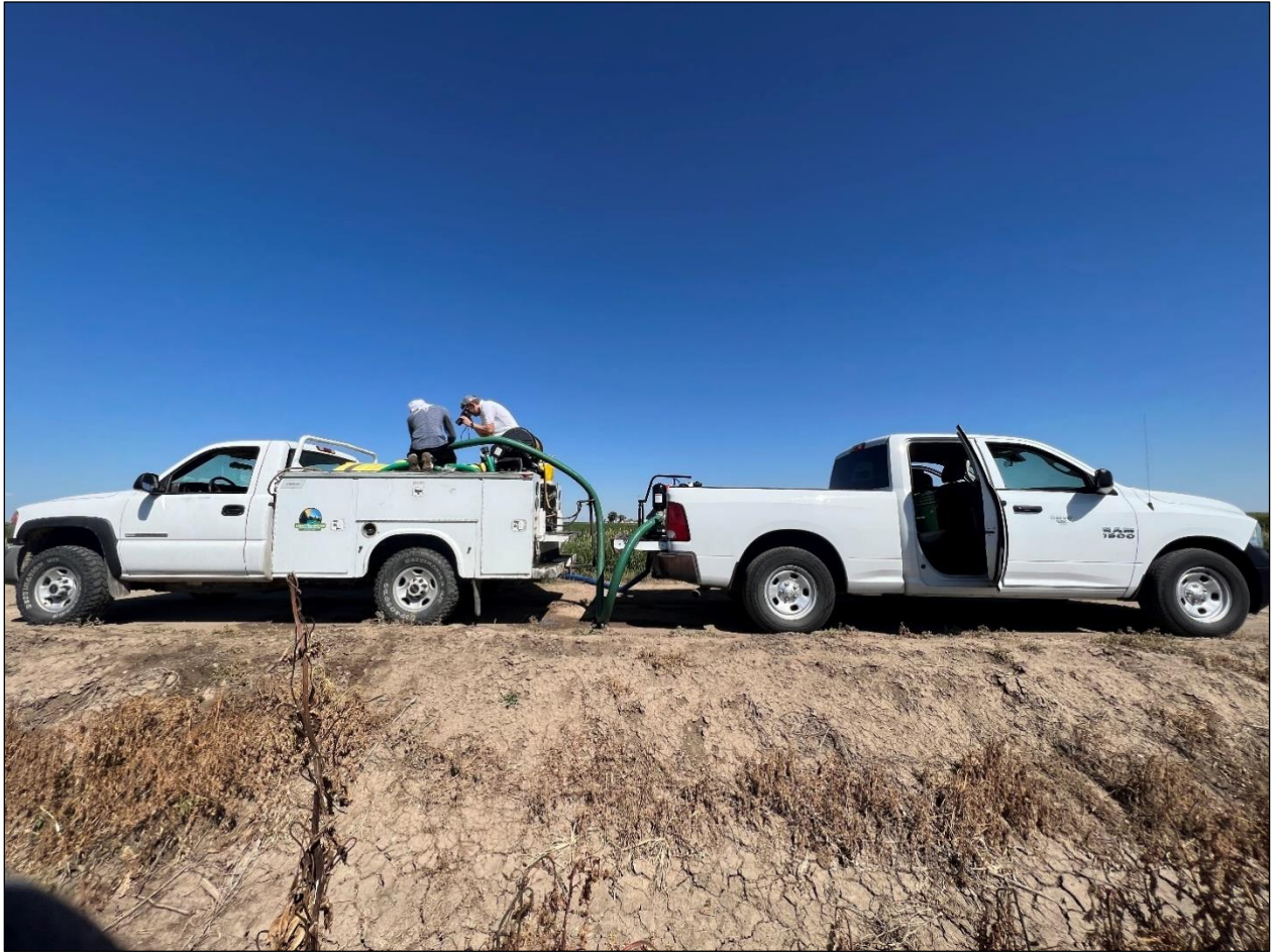
Figure B4-1: Wet Xanthan Gum application tools assembly. One truck carried the tank, while the other transported the generators and pumps.
