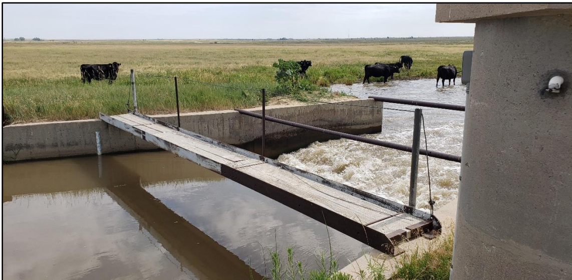
Figure B1-6: A view of a weri at the downstream end of the LWC canal in 2022. The downstream section of the LWC reach was located ~ 6-8 m upstream of this weir.
