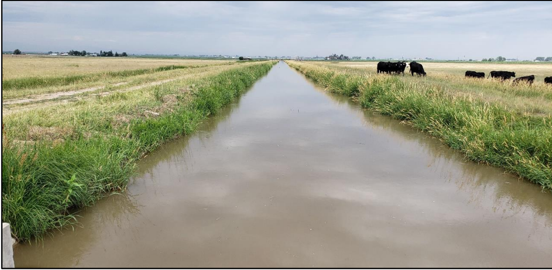
Figure B1-5: A view of the LWC reach from the downstream section looking in the upstream direction in 2022.
