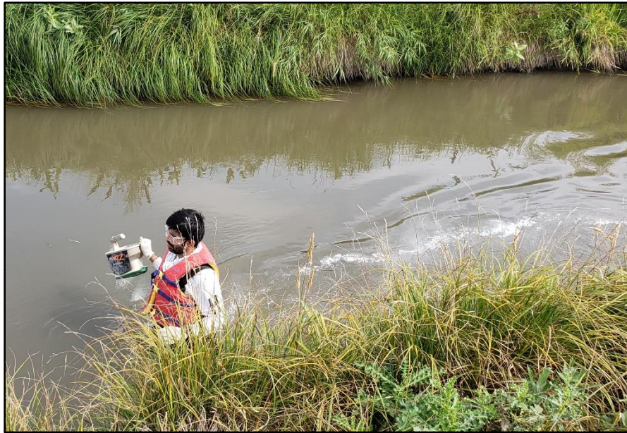
Figure B3-4: Technician applying dry Xanthan Gum in the LWC in 2021 using a handheld fertilizer spreader while walking in the canal.
