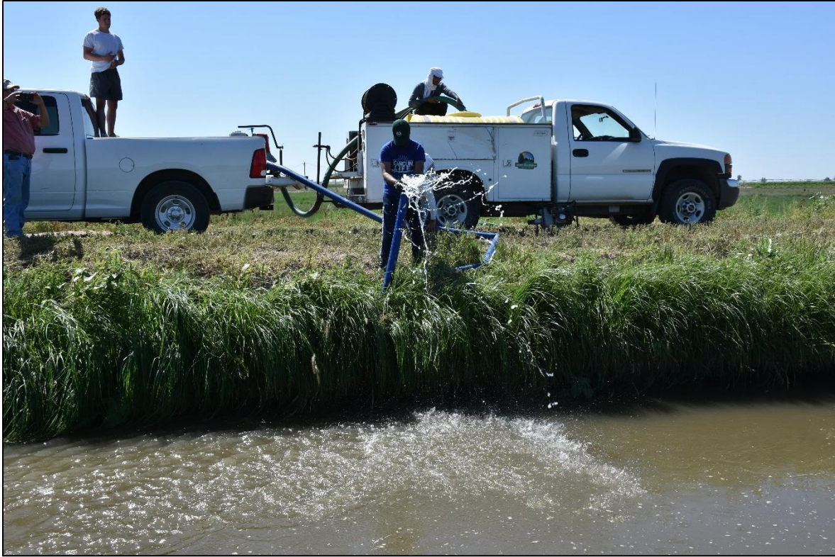
Figure B4-2: Technicians applying wet Xanthan Gum to the Larimer and Weld Canal from the bank, with the pump's throw covering the canal's width.
