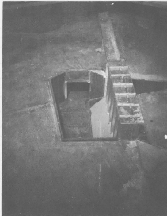
Fig. 6. Entrance to closed conduit
