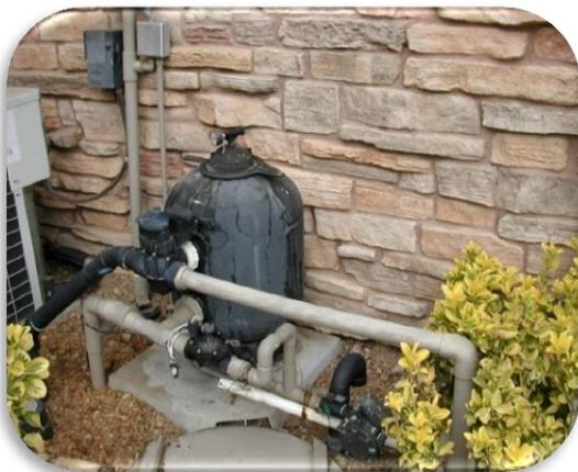
**Figure 3: ReWater® Graywater Reuse System for Irrigation using a sand filter**
