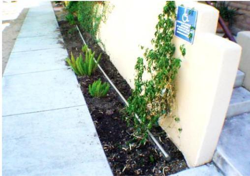
Figure 2: Drip Irrigation Utilizing Graywater
