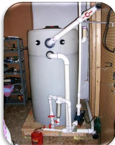
**Figure 4: Storage Tank for Subsurface Irrigation Graywater System**
