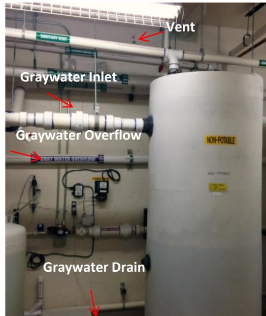
Figure 5: Graywater Tank and Components
