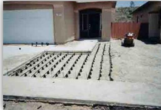
Figure 6: ReWater emitters (left) and emitters being installed under turf lawn for subsurface irrigation (ReWater®, 2014 [Link](#))
