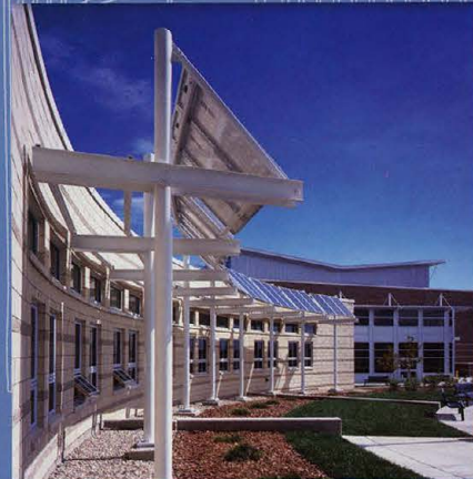
solar panels at fossil ridge high school, fort collins
