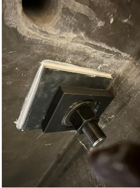
Figure 5.11 South side foundation bottom plate.
