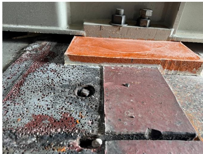
Figure 5.9 Foundation mounting pad (east side) with bolt.
