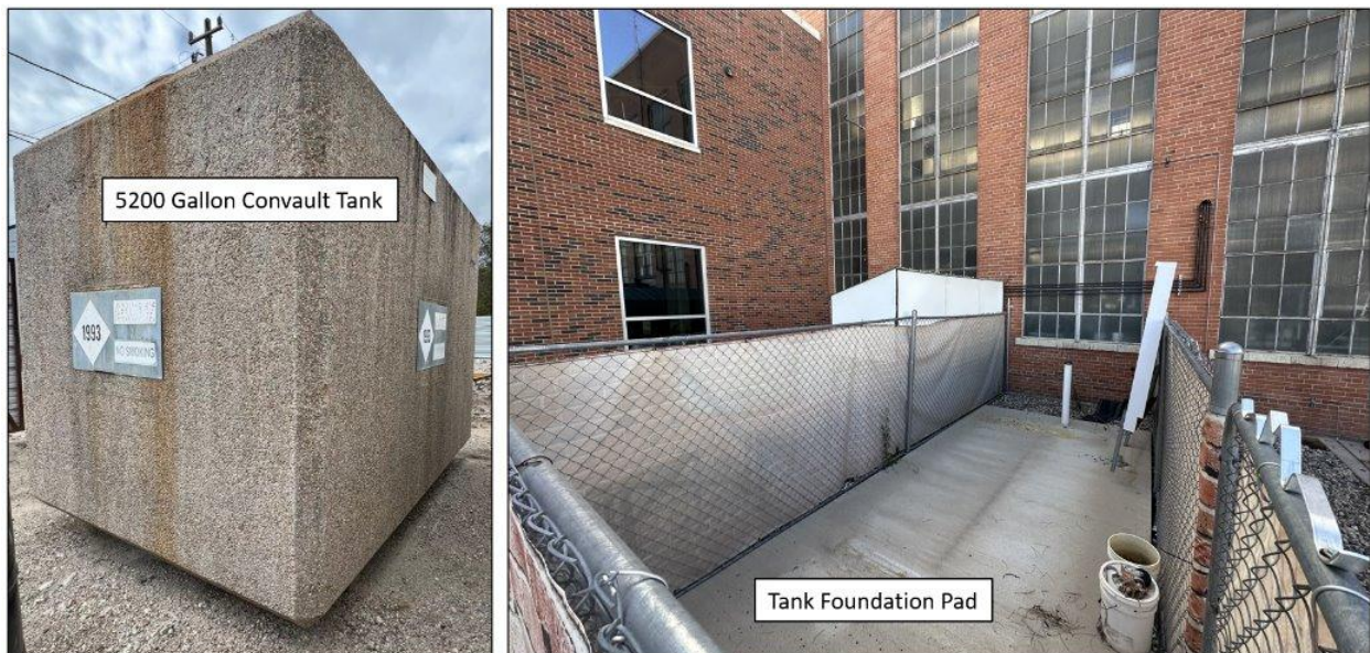
Figure 5.7 An image of 5200-gallon convault tank and foundation pad for the tank.
