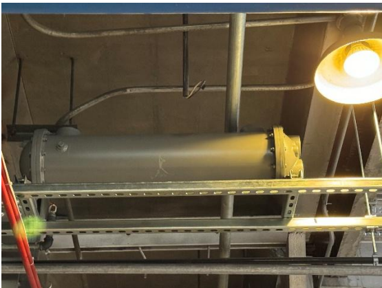
Figure 5.2 Heat exchanger for the lube oil system.
