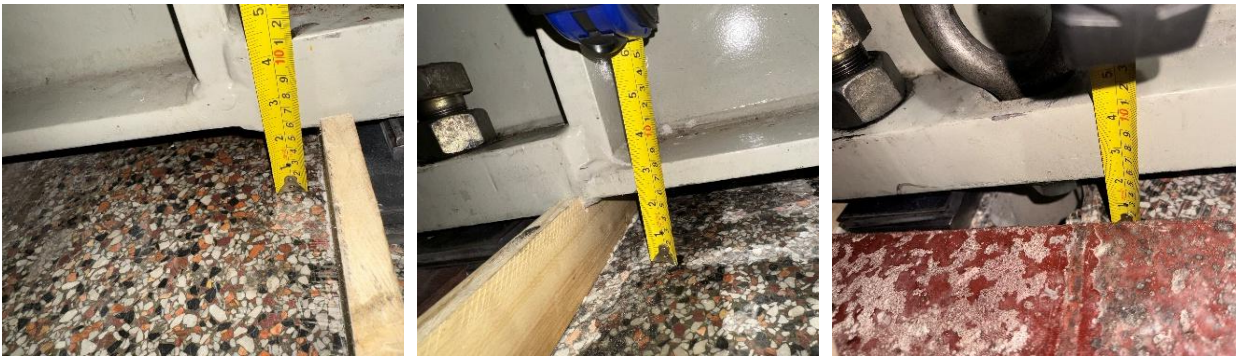
Figure 5.12 Foundation pad mold making.
