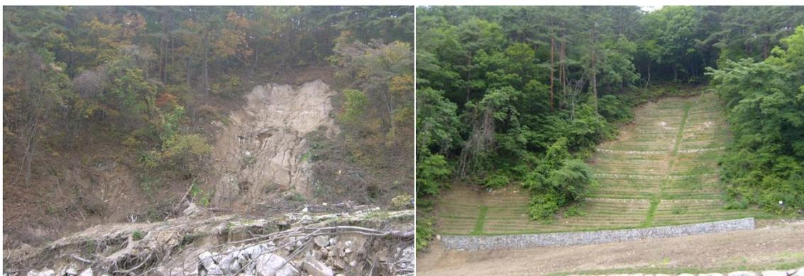
Figure A.1. Hill side control works example in Duksan Creek
