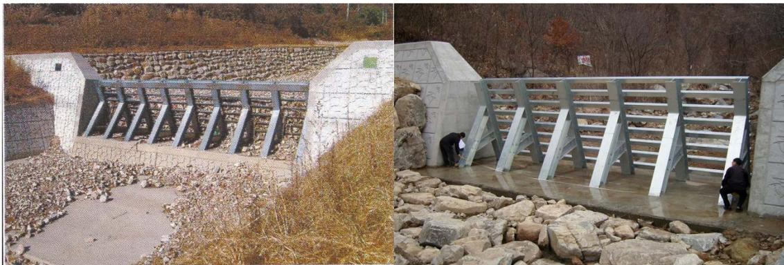
Figure A.4. Buttress dam example in Duksan Creek
