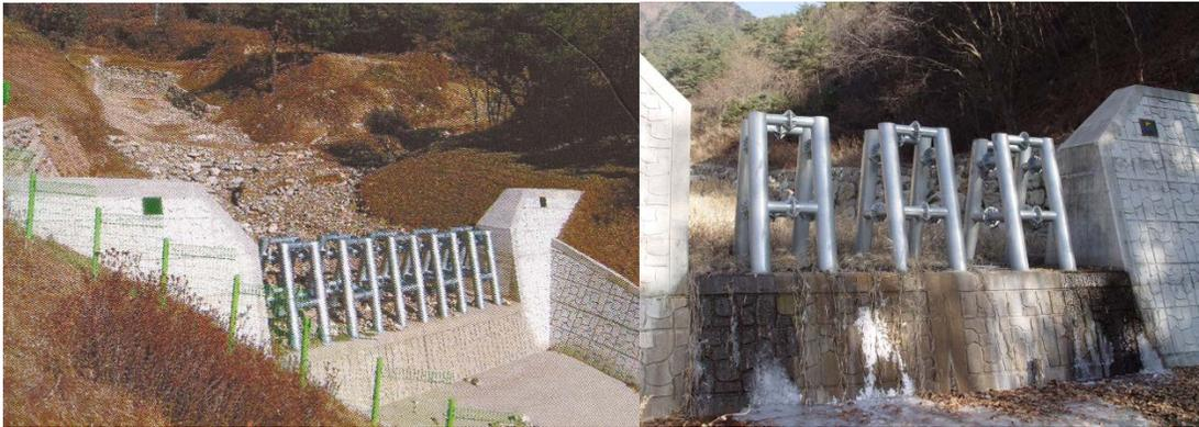
Figure A.3. Slit dam example in Duksan Creek
