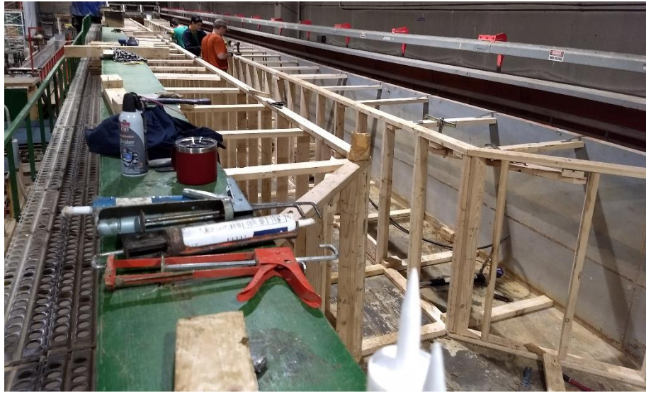
Figure 4.5. Construction of the wood frames supporting the sidewalls of the contracted channel. The view is looking into the entrance of the contracted channel; B_1/B_2 = 0.25 .
