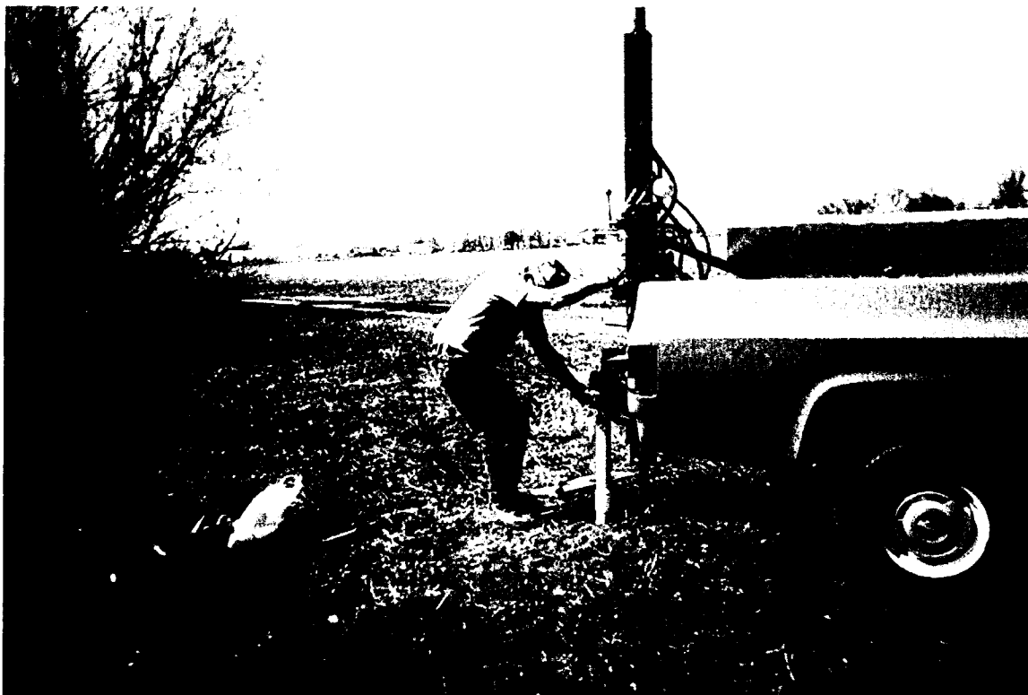
Figure G-12. Installation of Monitoring Well Adjacent to Edge of Irrigated Field
