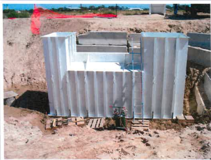
Figure 1. This image shows the retainer tank of the reference lysimeter after being set on the foundation. (Image courtesy of Lane Simmons)
