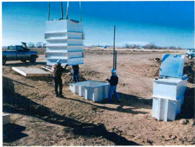
Figure 2. In this photo, the soil monolith tank is being installed in the retainer tank of the reference lysimeter. The monolith tank was set on the weighing mechanism inside the retainer tank. The manhole (right of photo) allows access to the underground chamber that houses the weighing mechanism, drainage tanks, and data loggers. (Image courtesy of Lane Simmons)
