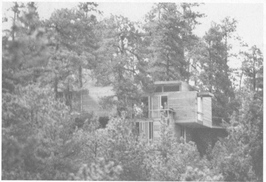
Poor access and heavy fuels provide no defensible space (see Issues C-11 page 32, and C-12 page 33).
