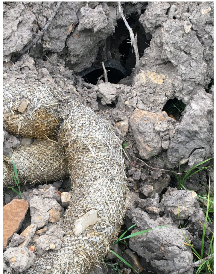
Figure 7: Materials fill in existing culverts on Sale #5. Photo: Diana Selby, CSFS
