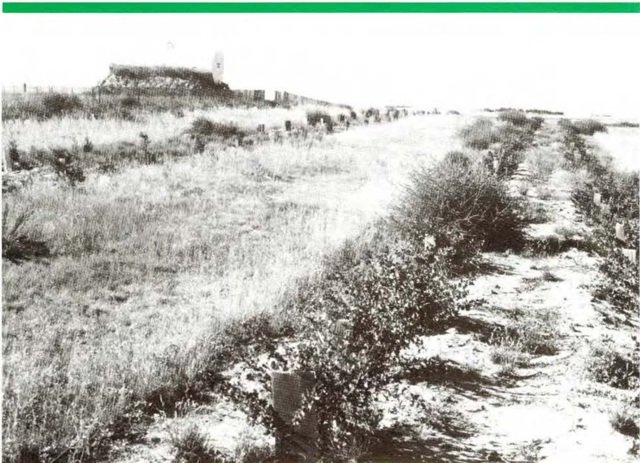
The drip system on this planting is fed from a 3000-gallon storage tank. The tank is elevated by placing it on a mound of earth.
