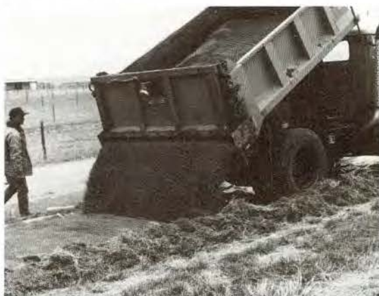
After seedlings are planted (top photo), plastic is laid and covered with gravel.
