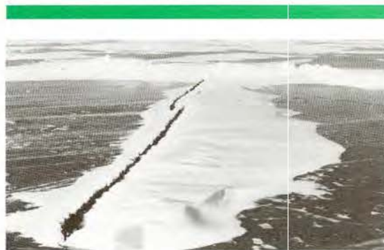
End effect means that considerably less snow is stored at the ends of a barrier.
