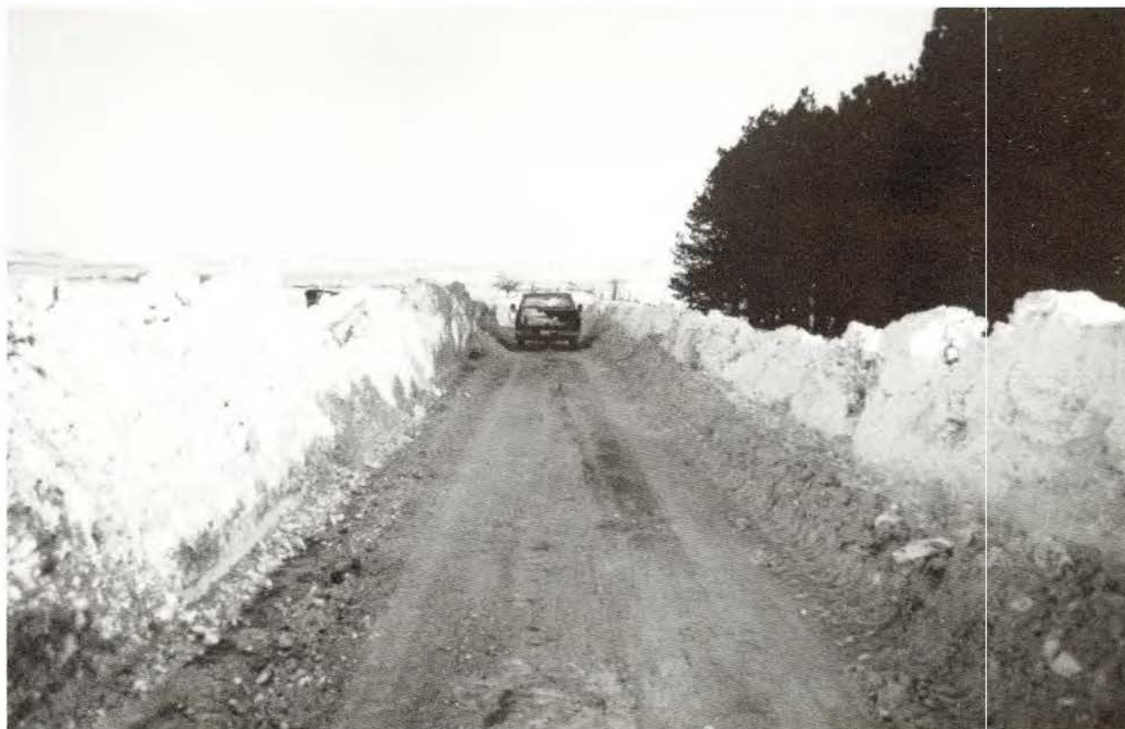
Barriers placed too close to the road result in excess drifting over the area needing protection.
