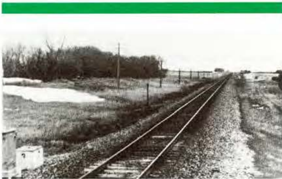
Recent photo of living snow fence planting established in the early 1900s along a railroad in North Dakota. Approximately 27 miles of such plantings still exist.
