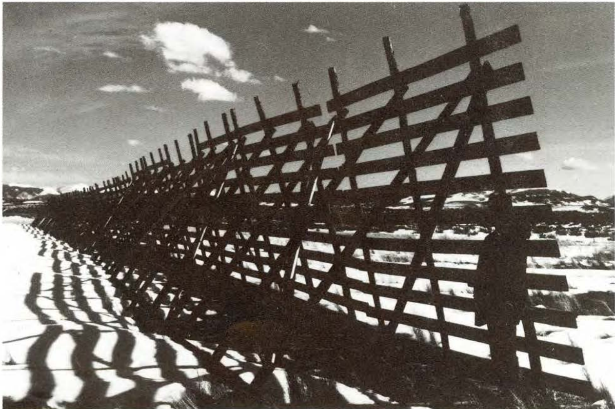
This Wyoming Design structure is 13.8 feet in height. With a porosity of 50 percent, it is very efficient in capturing and storing blowing snow.
