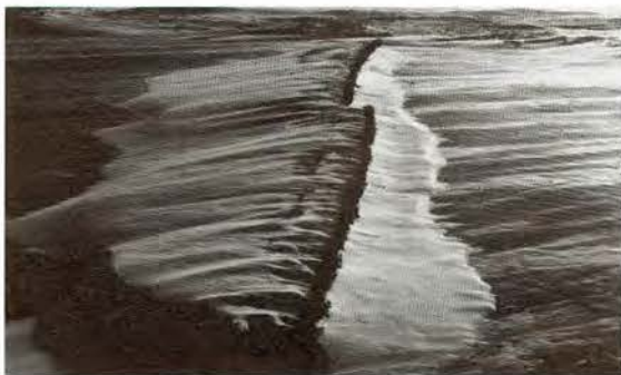
The portion of this barrier nearest the camera consists of two closely-spaced rows. Essentially, the leeward row becomes nonfunctional except to increase barrier density. In this instance, rows were about 20 feet apart.
