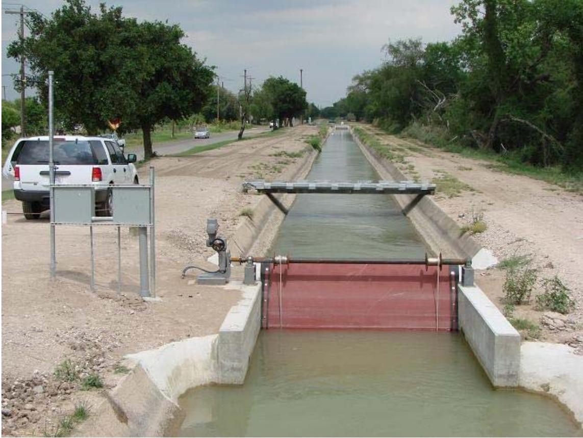
Figure 3. New radial gate and structure.
