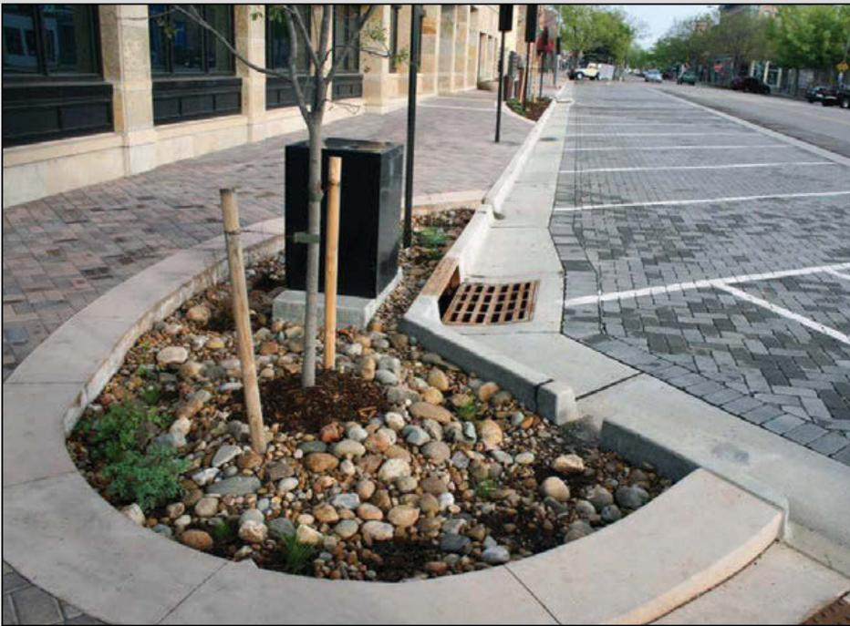
Figure 7. *Modular pavement and infiltration basin.*
