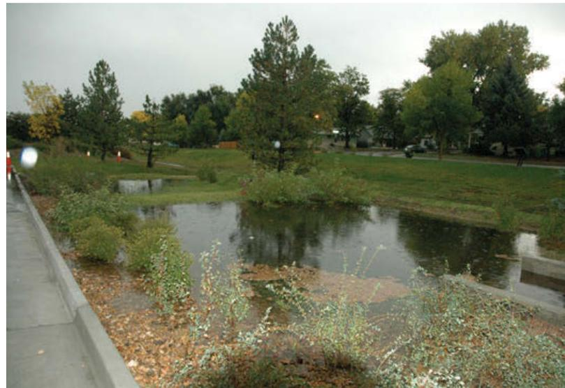
Figures 3 and 4. Bioretention cell installed in Fort Collins, CO during dry and wet weather. Bioretention cell treats stormwater runoff from an adjacent parking lot. Photos by Chris Thornton
