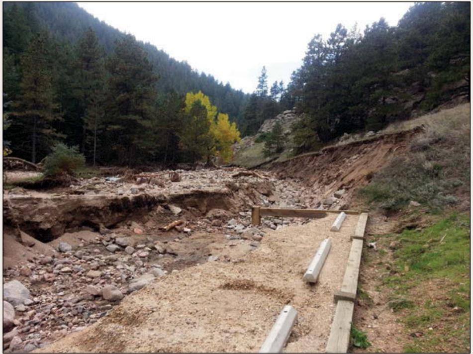
*New channel cut by Fourmile Canyon Creek in Boulder County near UDFCD border; Actual creek channel is left of photo. Damaged parking area served the Anne U. White Trailhead prior to the flood. Courtesy of UDFCD*
