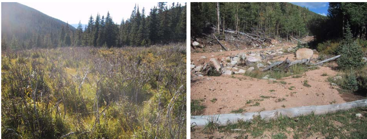
Figure 13. Sickly willows at the headwaters of Alamosito Creek where a road bisected a wetland (left), and large sediment deposit on the immediate edge of the creek (right).
