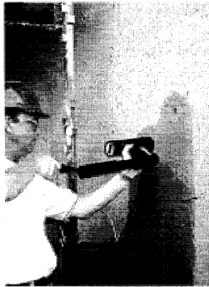
Figure 2.8: Testing for Strength with Pull-out Test of Fire Damaged Supporting Wall (Germann Instruments, 2006).
