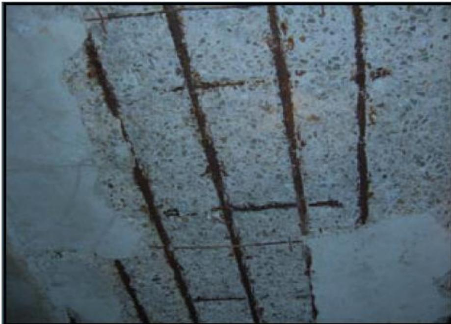
Figure 1.2: Concrete spalling due to corrosion (Feldmann 2008)
