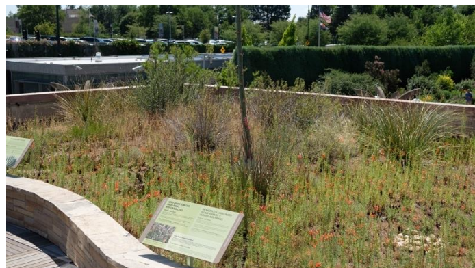
Figure 2. The extensive green roof site at Denver Botanic Gardens.
