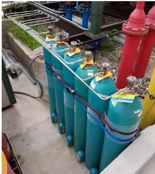
Figure 2-4. Ethane blending system setup.
