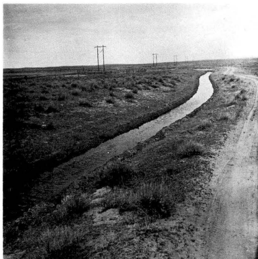
Photo 5. Sand Hill Lateral full of water from which recharge is occurring.
