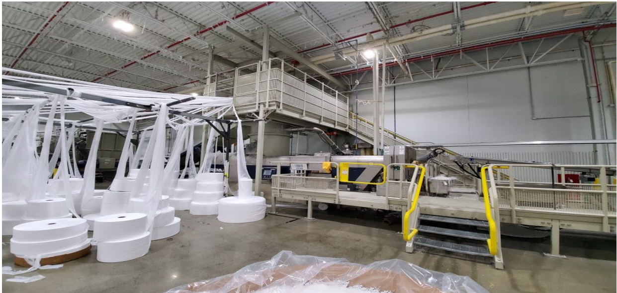
Figure 5.1 SMS Nonwoven fabrics being fed into the Erema Recycler. BERRY ©
