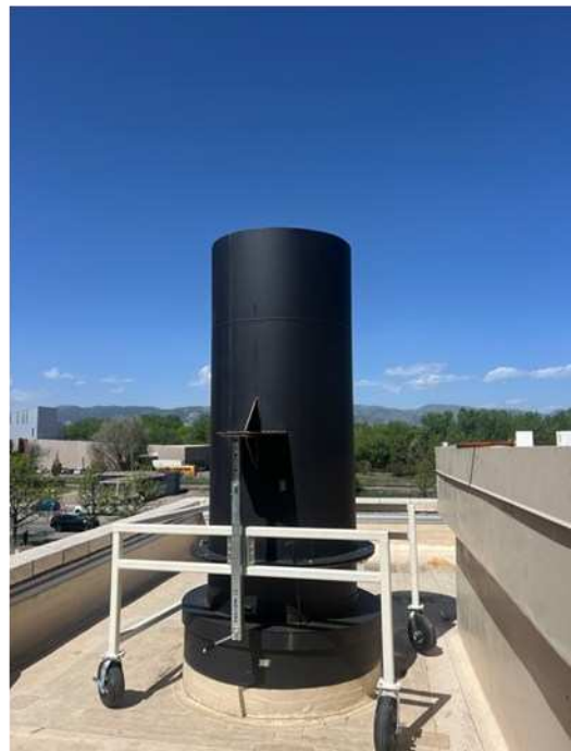
Figure 65: Mobile cart of raising and lowering exhaust stack view.
