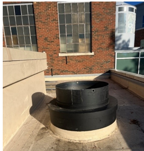
Figure 48: Completed installation of pipe extension and insulation thimble at roof.
