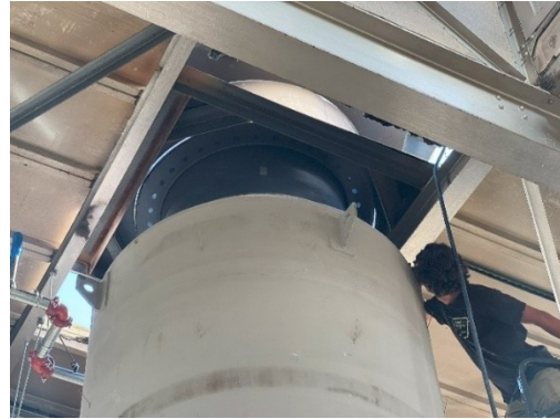
Figure 46: Decking and thimble installation process.
