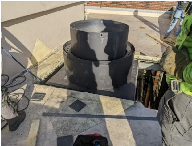
Figure 47: Thimble and pipe extension 2 installation process.
