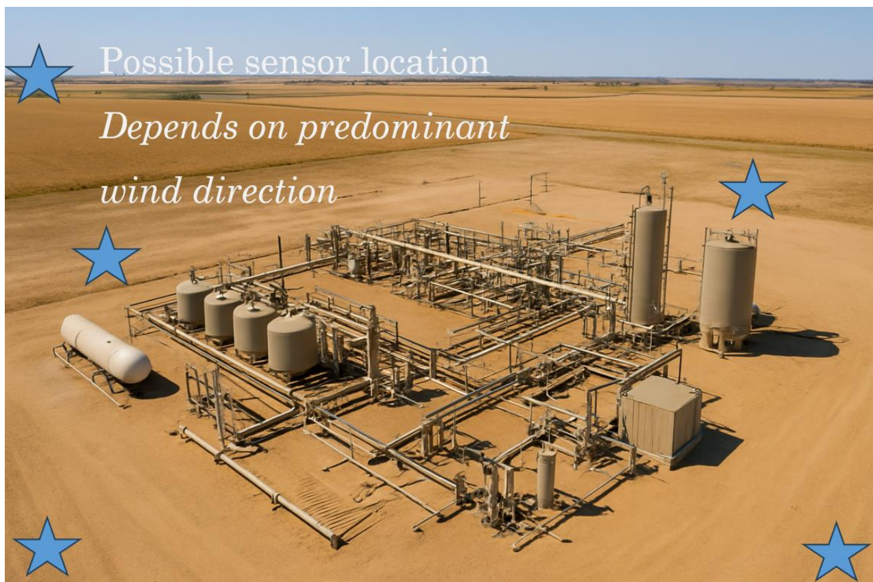
Figure 3. Sample configuration of continuous monitoring sensor deployment in an oil and gas facility (AI-generated image). Source: Created with ChatGPT (2025) based on concept adapted from Herrick (2019).
