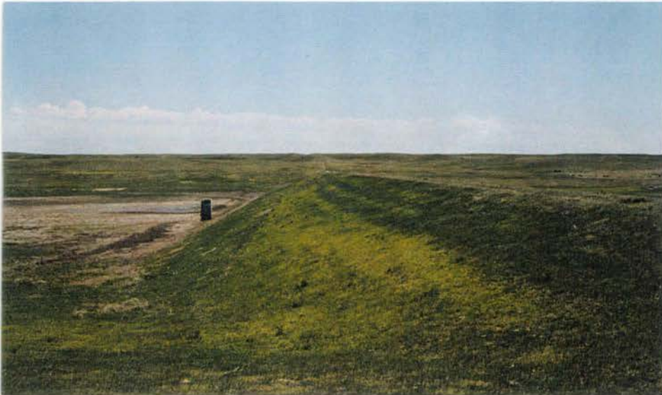
Figure 1.2 - View looking east across upstream face of floodwater retarding dam SS-3.
