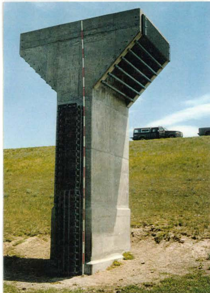
Figure 1.3 - Inlet tower on upstream face of floodwater retarding dam SS-5.
