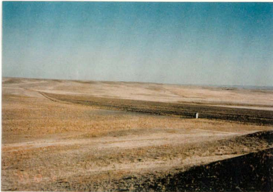
Figure 6.7 - Dam SS-3 under dry conditions on Dec 4, 1997.
