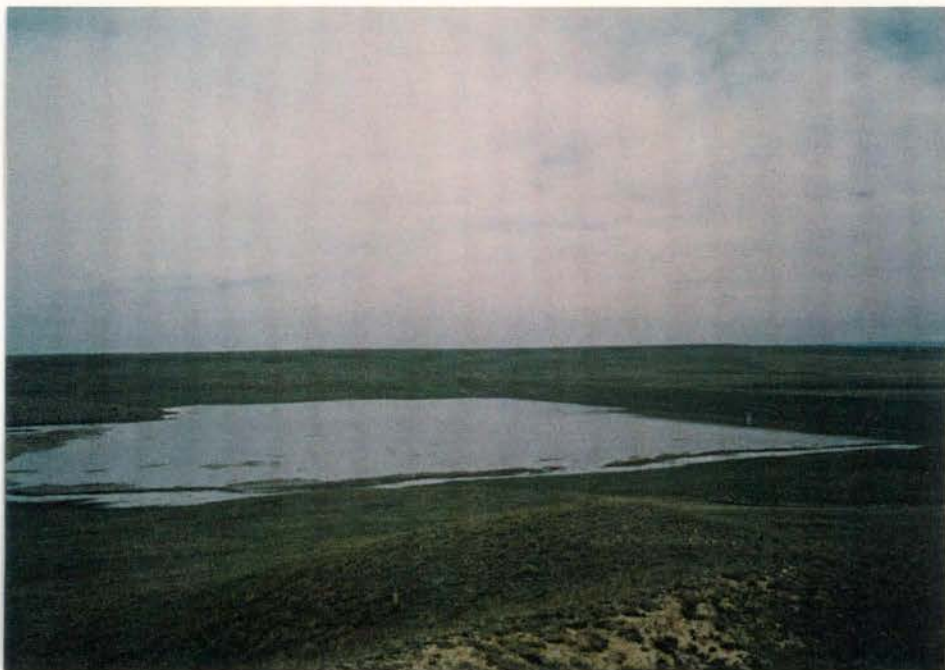
Figure 6.8 - Dam SS-3 after storm on June 11, 1998.
