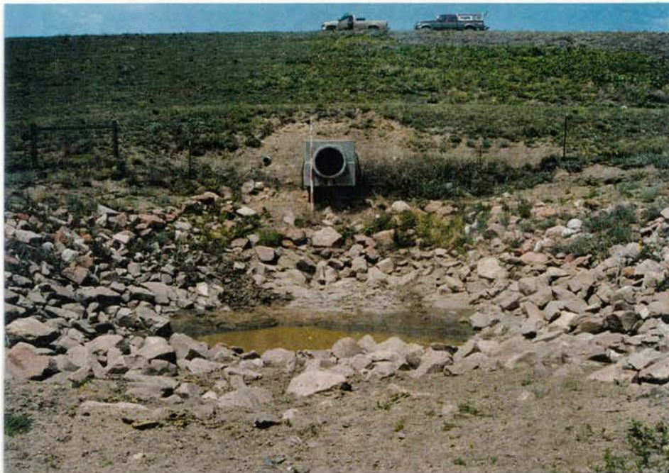
Figure 1.4 - Outlet works of floodwater retarding dam SS-5.
