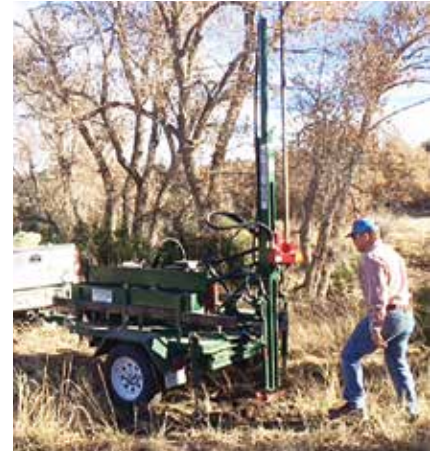
Drilling shallow alluvial groundwater wells. Photo by Blake Osborn.
