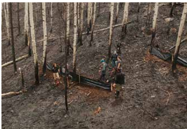
CSU students helping install sediment fencing on severely burned hillslopes. Photo by Blake Osborn.
