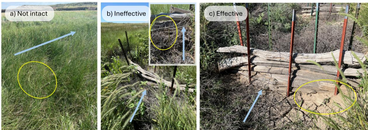
Figure 6: Categorization of log-based erosion control structure outcomes. Blue arrows indicate flow direction.
