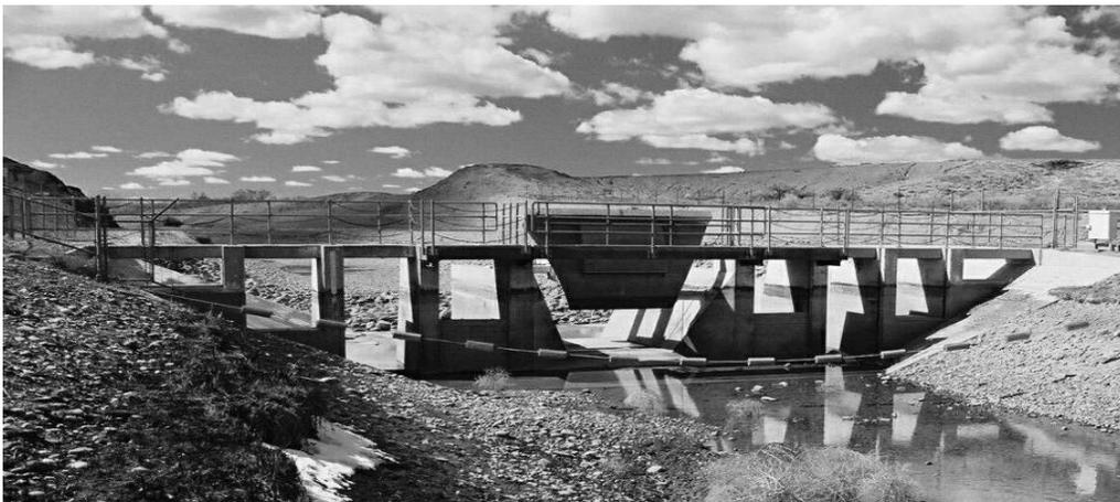
Figure 4. Amil Gate / Stop Log Structure
