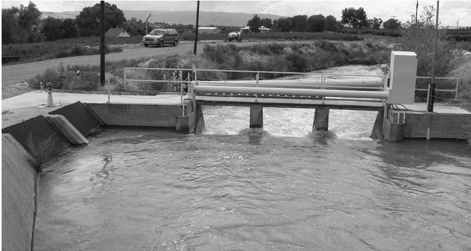
Figure 3. Gate Installed in Modified Stop Log Structure
