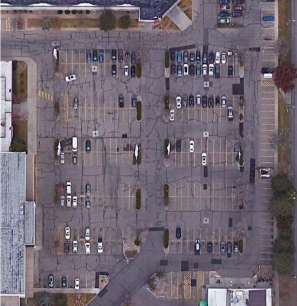
Figure 2.4.1b: An example parking lot from the General Commercial District and Employment District study area from census block #80690010071. Here, we can see that many of the landscaped islands are treeless, even though Fort Collins Municipal Code calls for tree cover (Satellite imagery by Maxar Technologies 2023).
