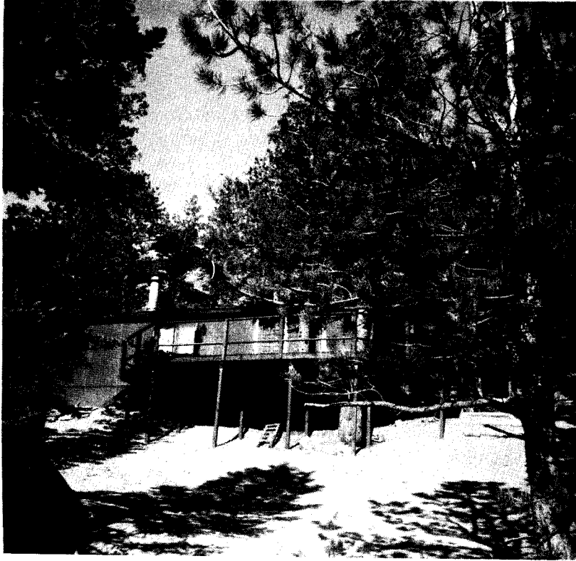
Figure 9. Cabin Served by the Full Scale Unit.
