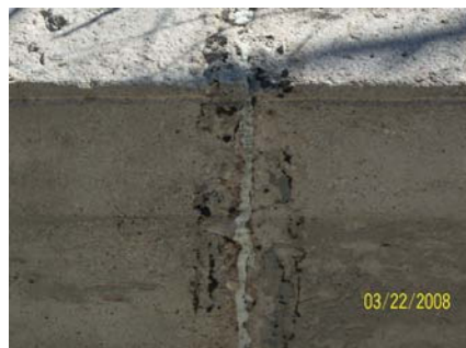
Example of patch peeling away
