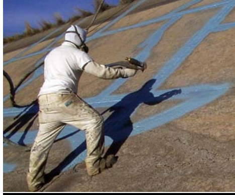
AquaLastic® being applied using high pressure application equipment
