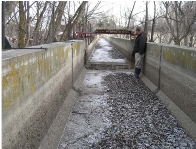
Degraded high level flume photographed early spring '08
