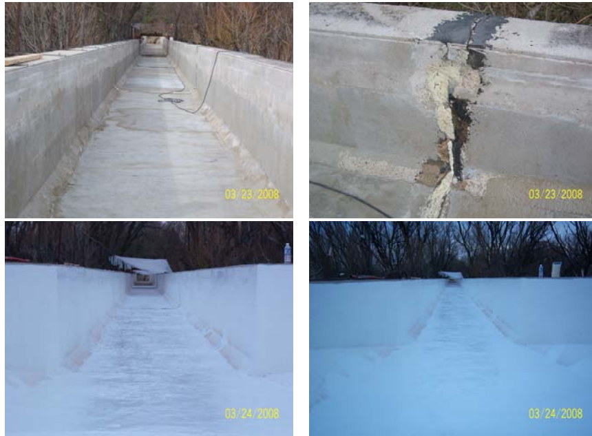
Several processes took place before AquaLastic® was applied
