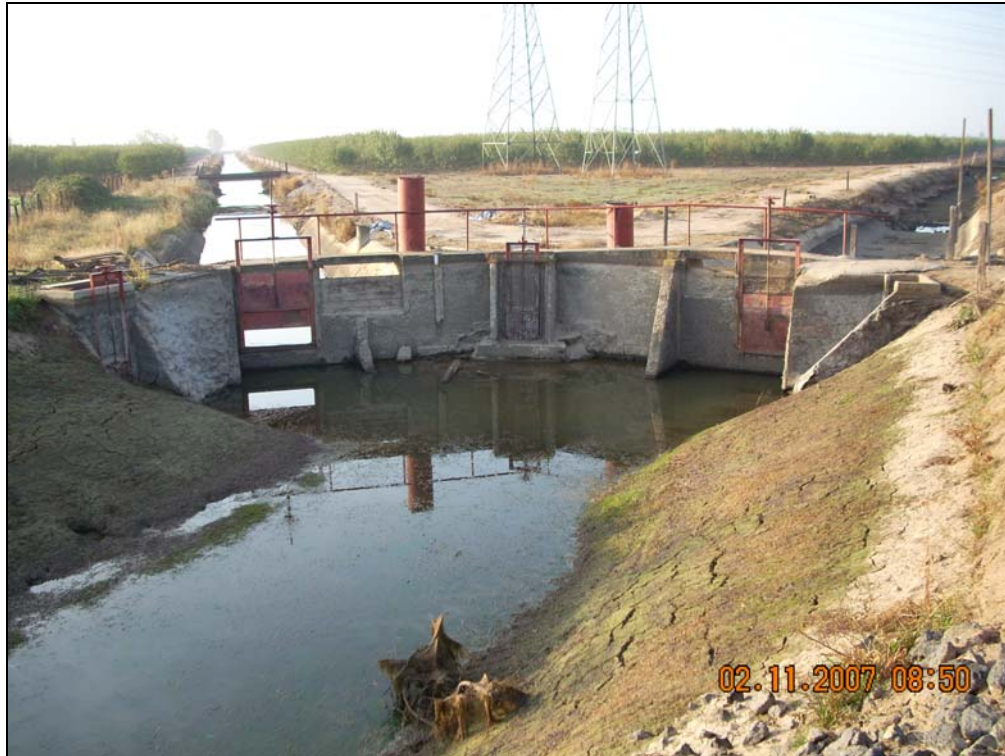
Figure 3. OID Diversion Structure Pre-Modernization
