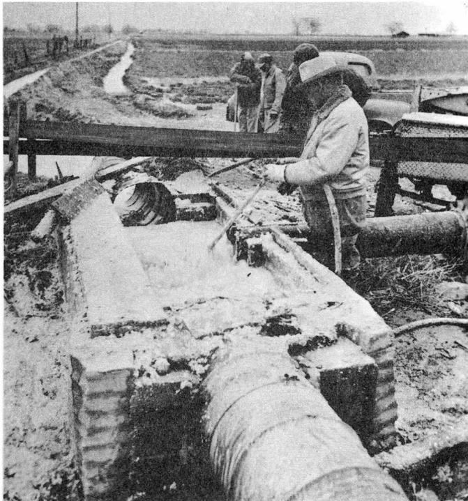
Fig. 1 Air jetting into a small continuous flow using the stilling basin of the pump as a mixing pool.
