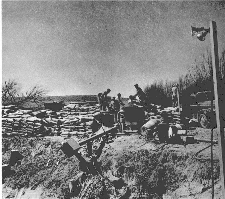
Fig. 2 Metal 9-in. Parshall flume used to determine inflow.
