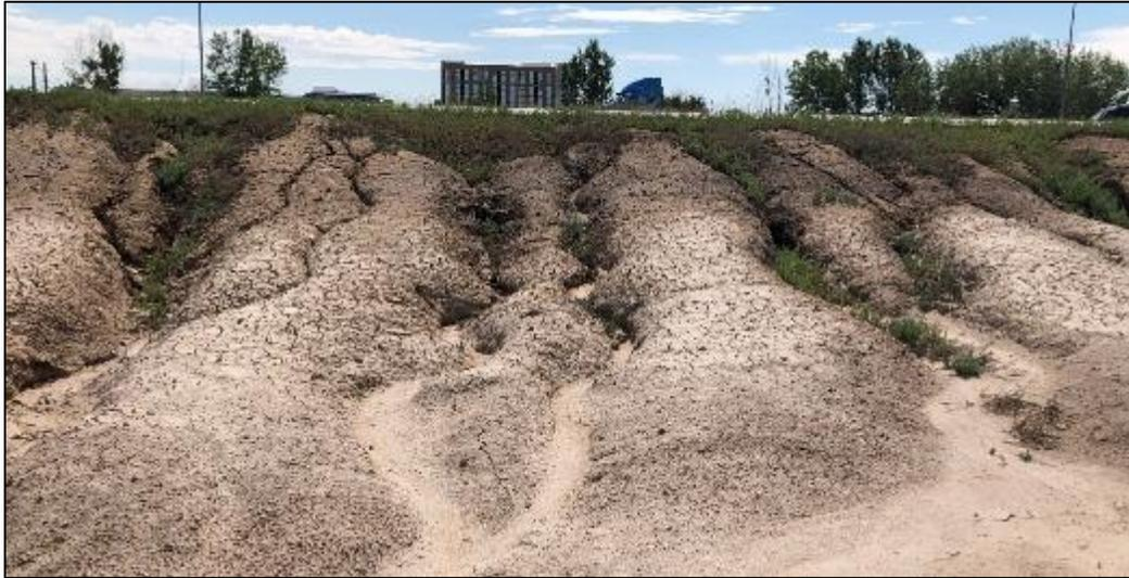
**Figure 4.** Southbound PBTC roadside. Extreme gullies created by water runoff from the road. No vegetation, aside from kochia, due to  $MgCl_2$  and water erosion.
