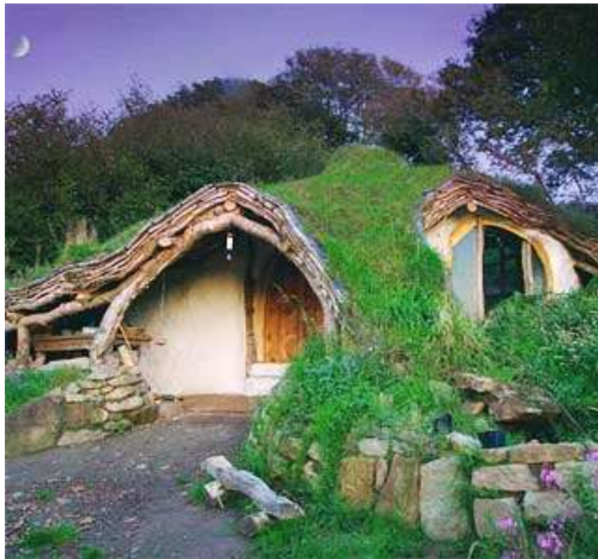
Figure 29. Earth Homes Now. A photo of a built environment sharing exterior walls with natural earth. Earth sheltered homes.
